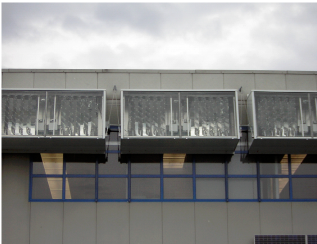
Fig. 5. Collectors concentrate the sunlight into light guides for distribution within the building.
