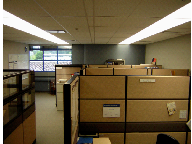
Fig. 6. The original prismatic troffers were replaced with dual-function light guides.
