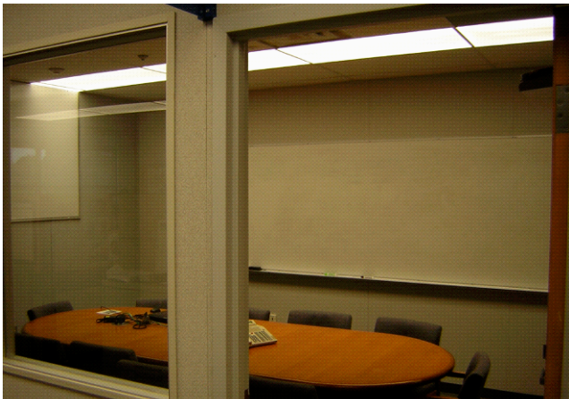
Fig. 14. The guide delivers sunlight into a windowless conference room.
