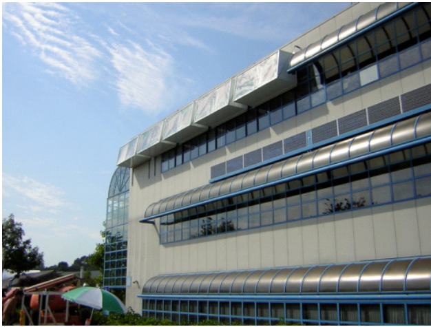
Fig. 4. Collection modules installed at BCIT's
