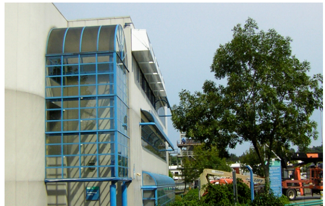
Fig. 7. The canopies also provide shade for the windows below, reducing glare and air conditioning cost.
